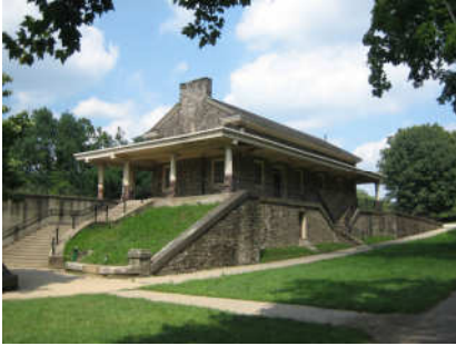
Trains no longer stop at Valley Forge, but the structure provides ample space for orientation. Soon it will become a visitor contact station.
