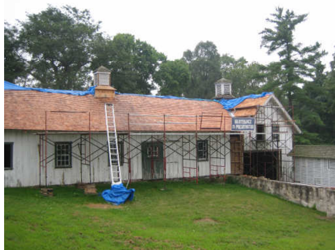
Re-roofing historic structures is an essential step toward their stabilization.
